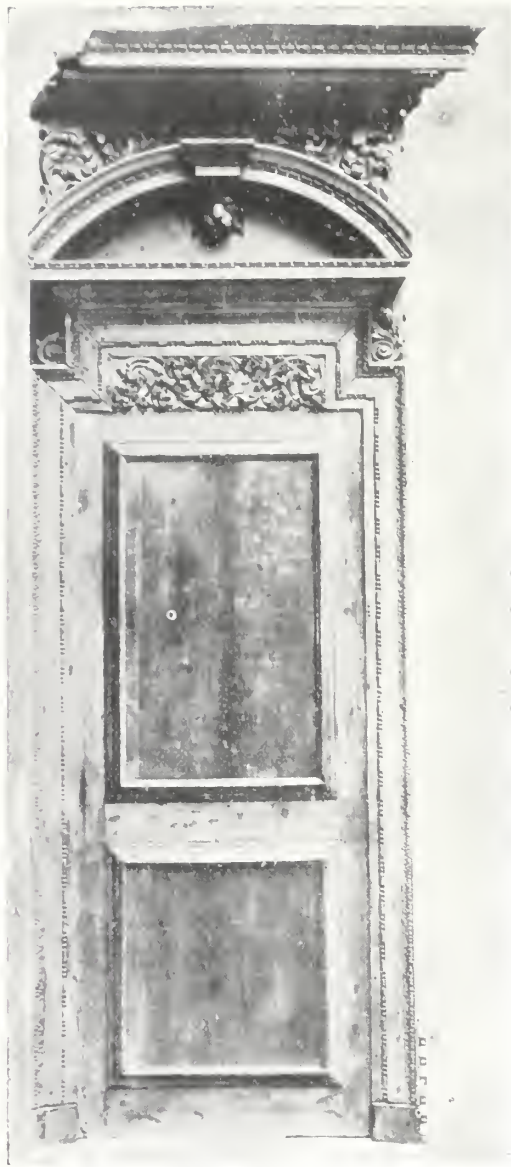
DOOR, PART OAK, PART CEDAR FROM NO. 5, CLIFFORD'S INN AN OLD HOUSE ERECTED BY JOHN PENHALLOW, 1680-8
